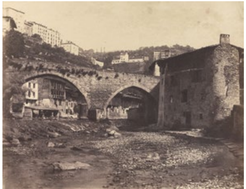
André Giroux. Le Pont de Seychalles sur la Duralle, Thiers, Puy de Dôme , salt print, c.1855. "This photograph has the finest registration of detail of the all photographs in this exhibition, capturing all the subtleties of light and shadow."
